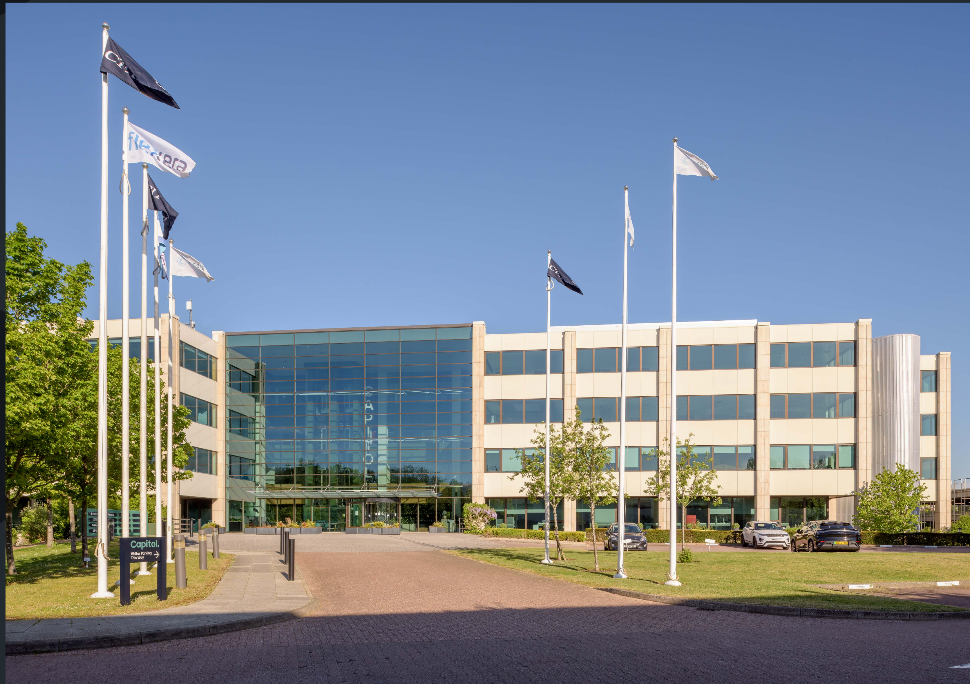
Building exterior and main entrance
