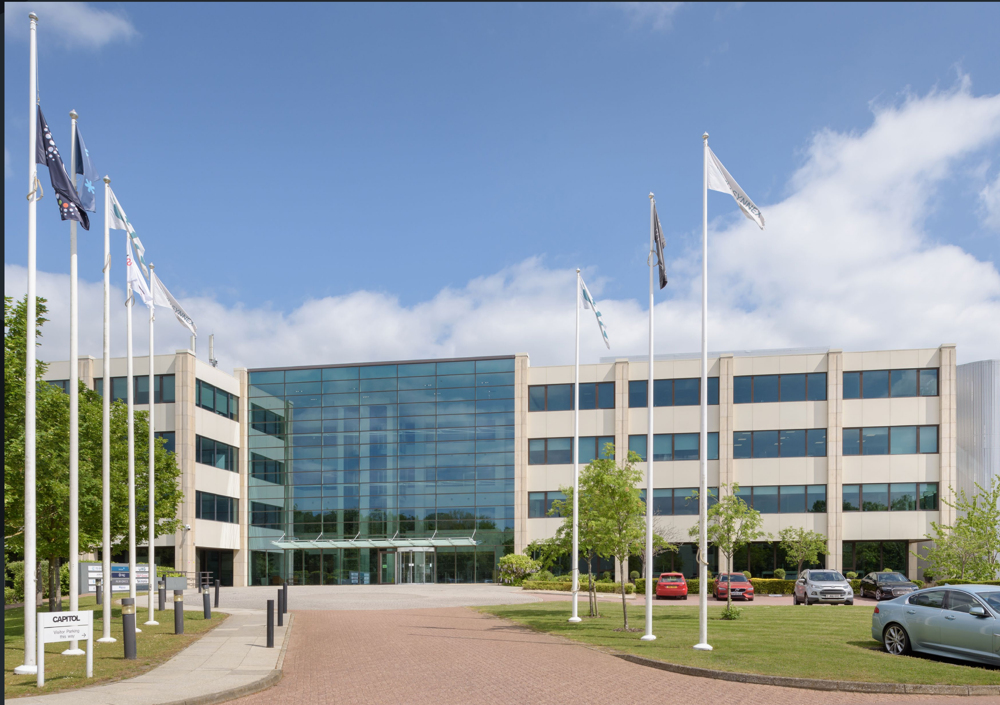
Building exterior and main entrance
